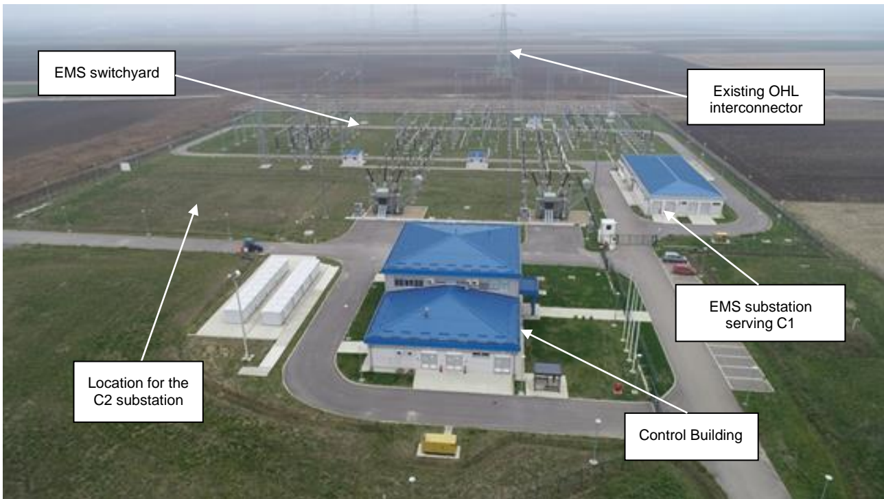
Figure 7-1 Čibuk Control Building Compound
