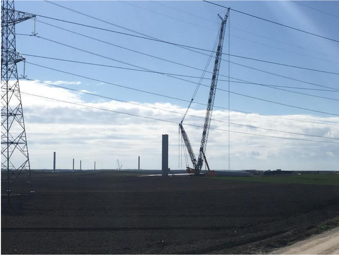
Figure 5-18 Erection of the first tower section
