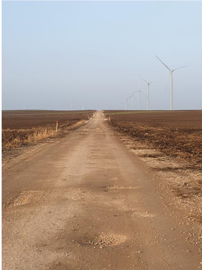
Figure 5-3 Čibuk 1 Access Track and Turbines
