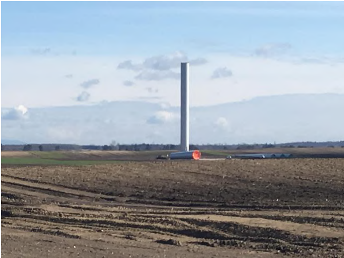
Figure 5-19 First tower section installed
