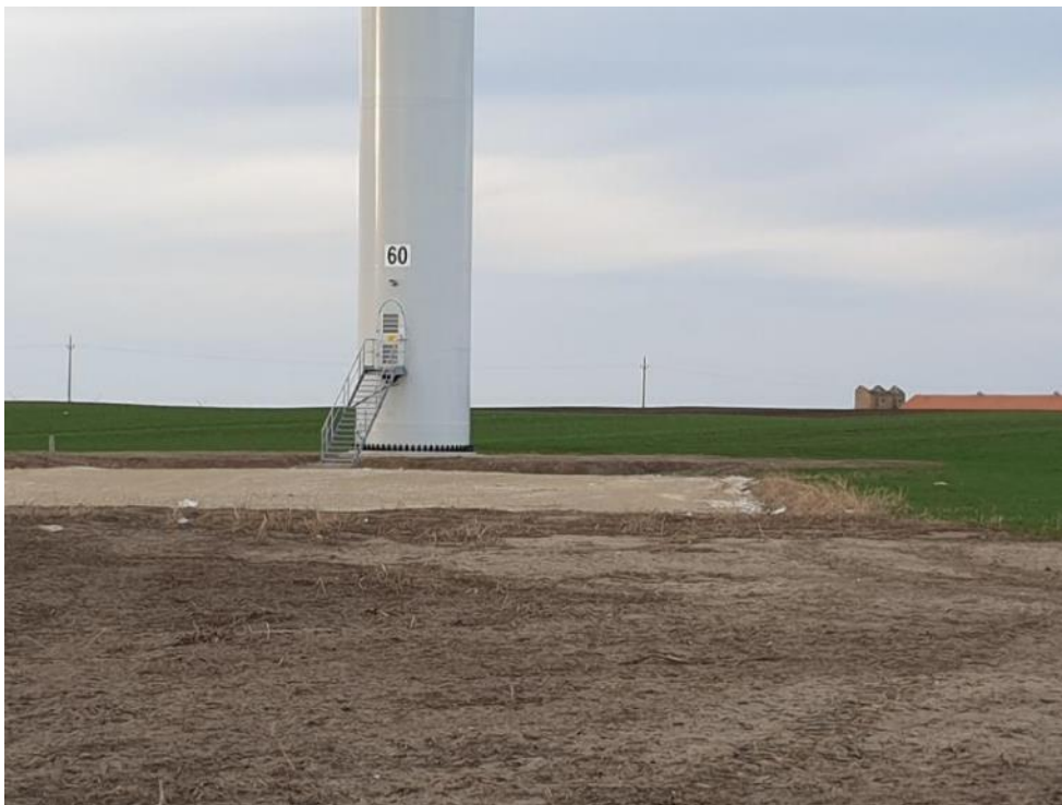
Figure 5-4 Čibuk 1 WTG 60 with its maintenance pad
