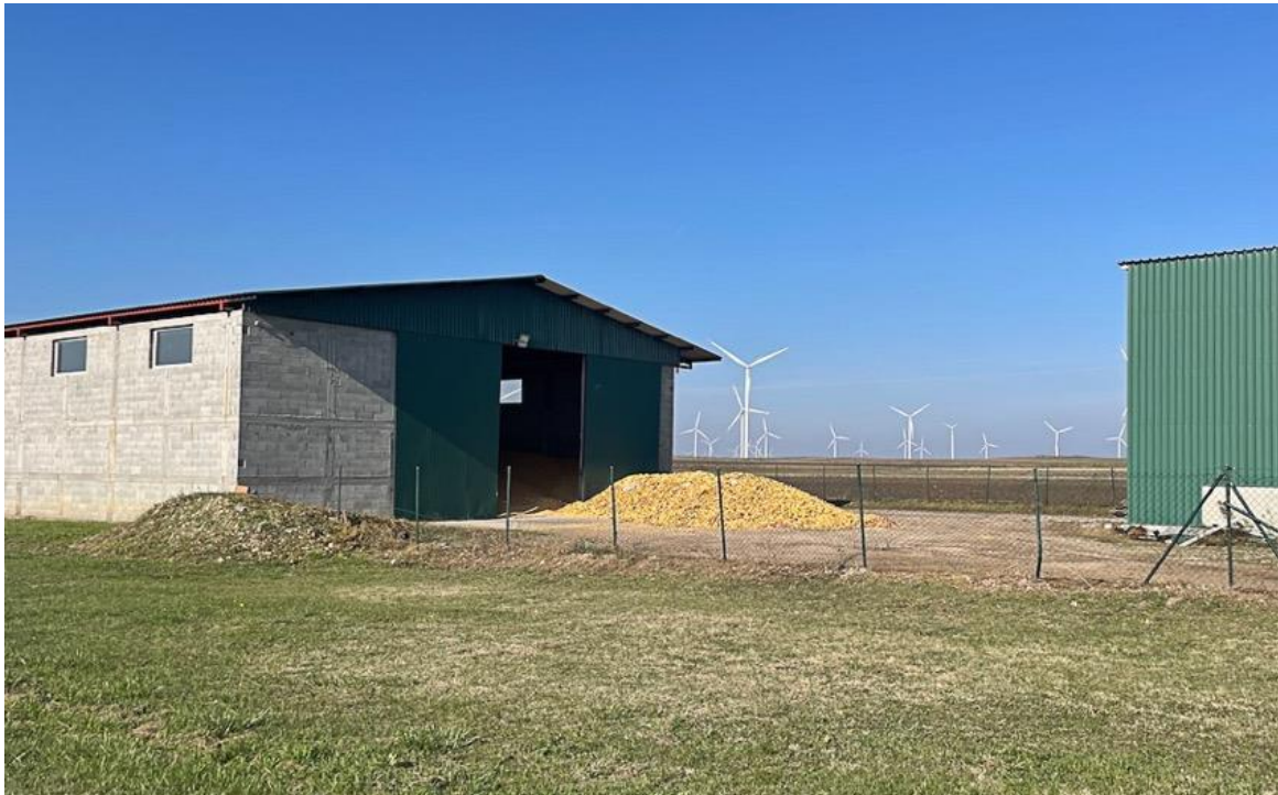
Figure 7-4 Crop Warehouse in the North-Eastern Portion of the Site
