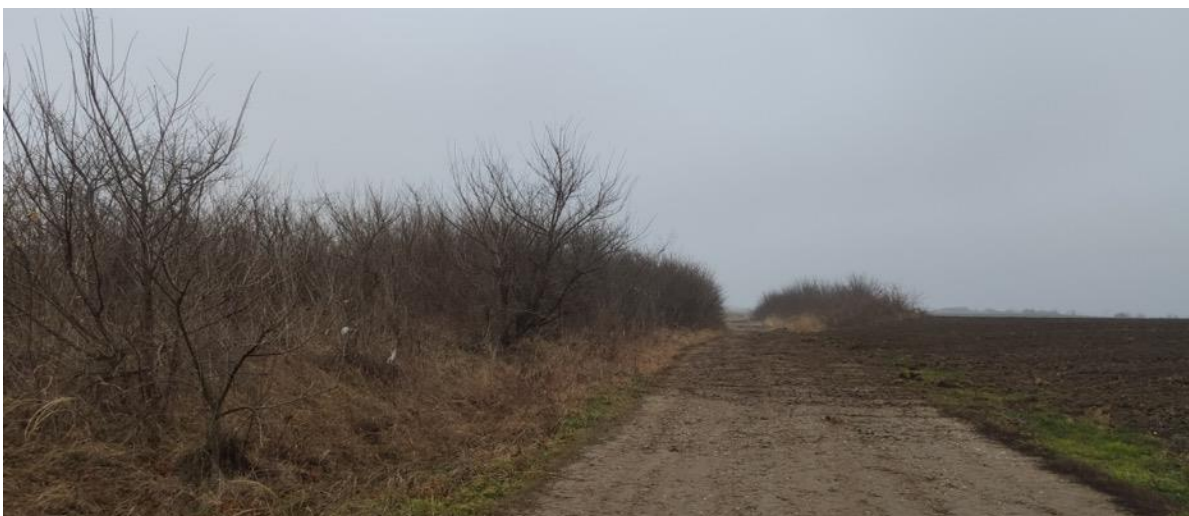
Figure 7-20 Deliblato Road is Paved with Crushed Stone and with Linear Scrub Vegetation Along
