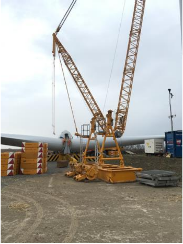
Figure 5-21 Preparing the nacelle and blades to lift
