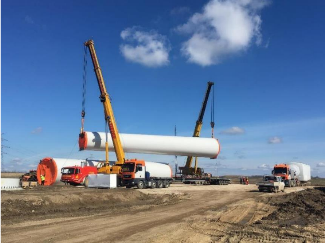
Figure 5-16 Off-loading a tower section from the delivery truck
