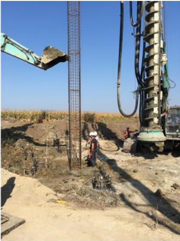
Figure 5-14 Forming the WTG Foundation Pile
