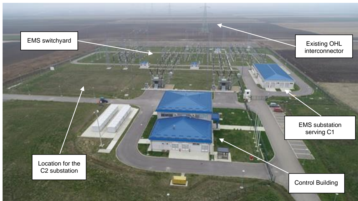
Figure 1-4 Čibuk Control Building Compound
