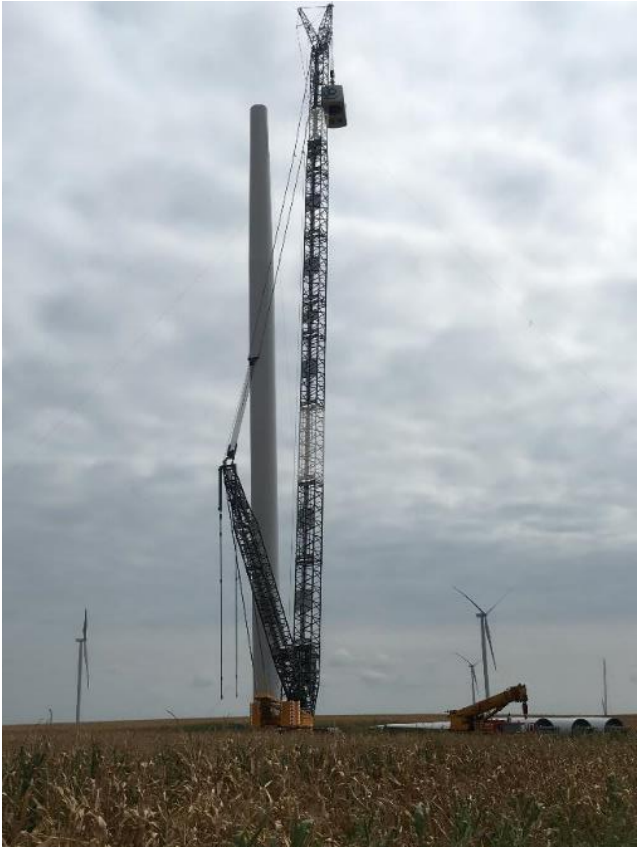
Figure 5-20 Second and third tower sections installed
