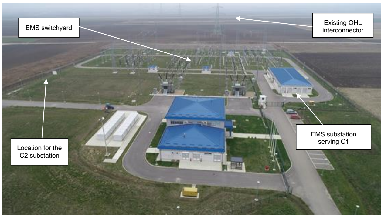
Figure 5-12 Čibuk Control Building Compound
