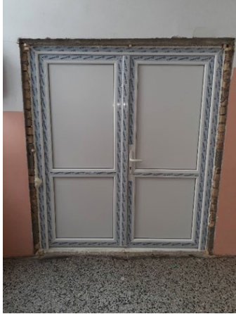
Above: Door replacement in Elementary school Sava Maksimovic
